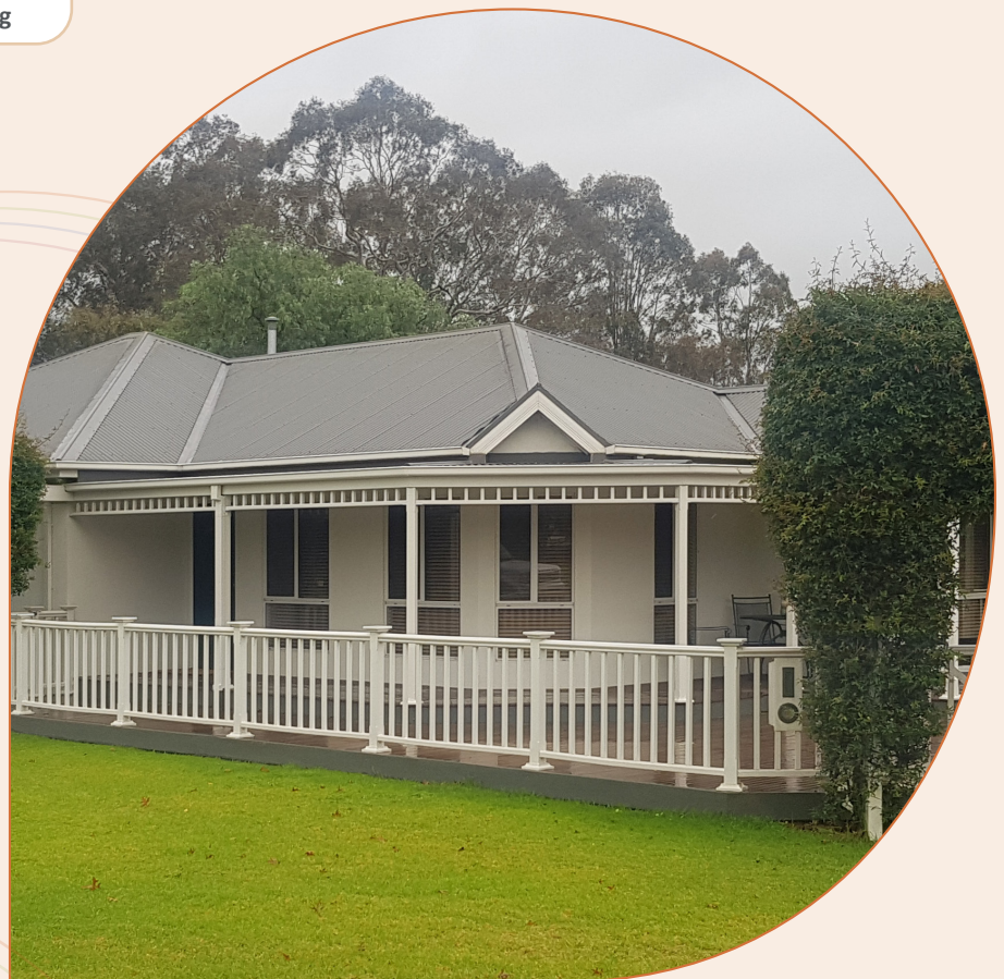
Residential Property in Maffra
